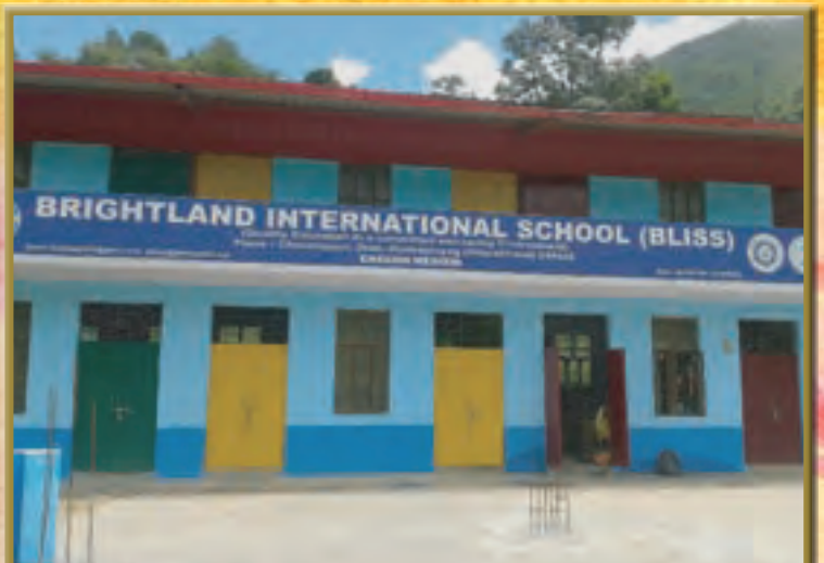
DSF's rebuilds a school in Rudraprayag, Uttarakhand that had been destroyed in the 2013 floods.
