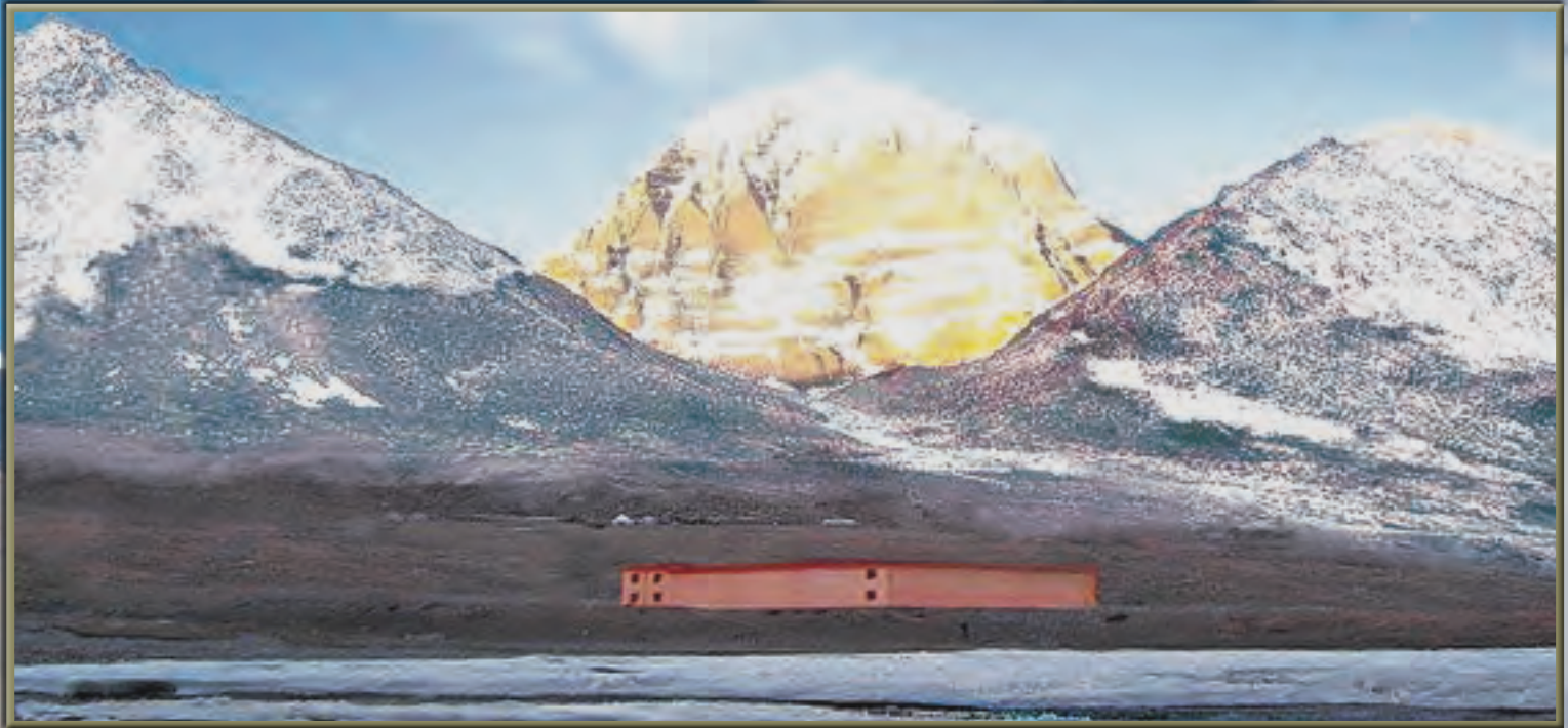
Rear view of Parmarth Mansarovar Ashram, Dirapuk. All rooms in the ashram face Mt. Kailash
