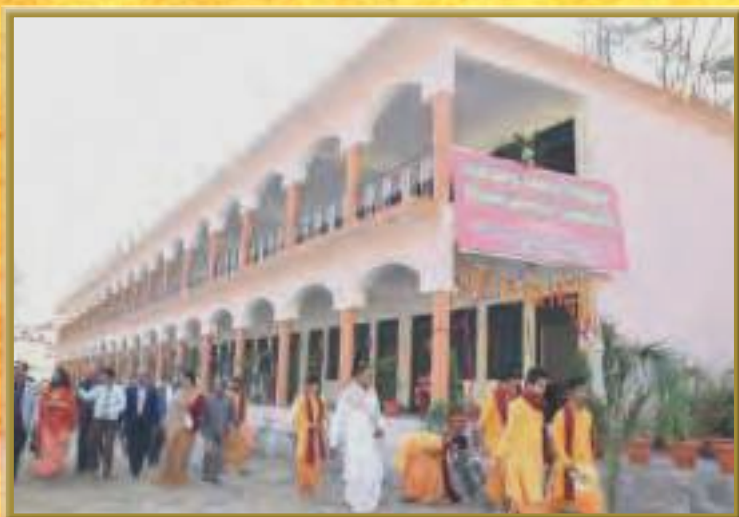
Inauguration of DSF's newly constructed skills training centre, in joint partnership with the Paropkar Sansthan, in Uttarakashi, Uttarakhand that had been washed away in the tragic 2013 floods.
