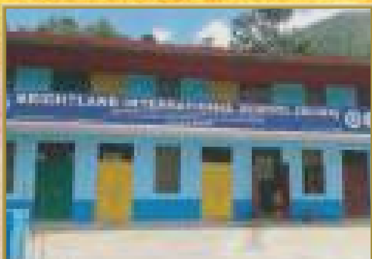
DSF's rebuilds a school in Rudraprayag, Uttarakhand that had been destroyed in the 2013 floods.
