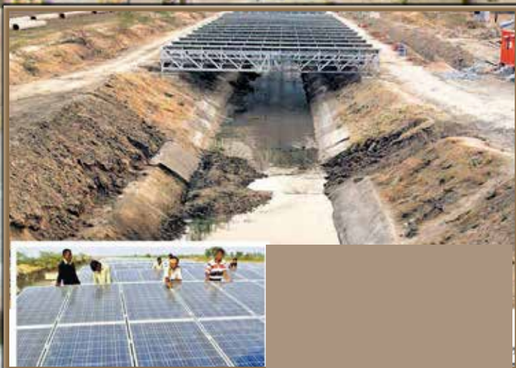
Solar panels over a canal in Gujarat prevent evaporation of precious water, whilst producing energy and saving land for other uses
